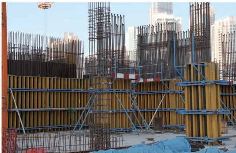
The column formwork can also be used in the concrete pouring of inclined column.
